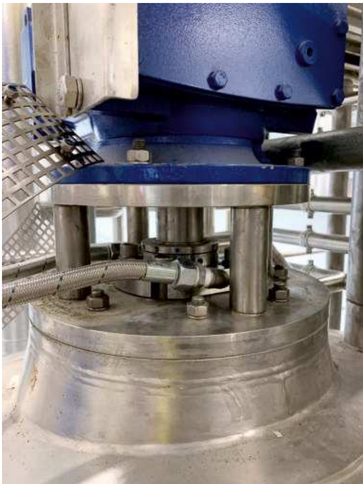
Double - Cartridge type 922CX according to API Plan for drug production
